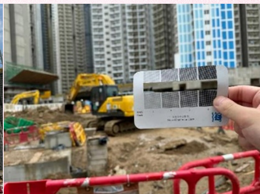
Inspection of emission by construction plants to ensure no excessive dark smoke is emitted 檢測施工機械以確保沒有釋放過量黑煙
