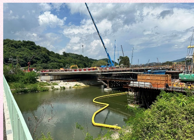
Install silt curtains to protect the river from leakage of silty water 設置淤泥屏障，以保護河流免受泥水滲漏影響
