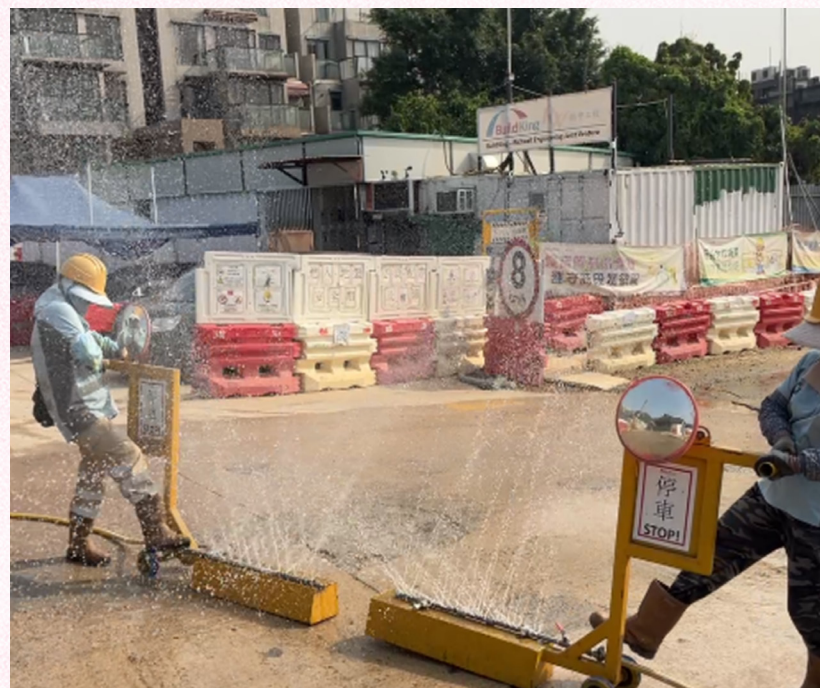
The wedge prevents the vehicle from sliding, hence also improving the efficiency of wheel washing 此楔塊能防止車輛滑動，從而提高清洗車輪的效率
