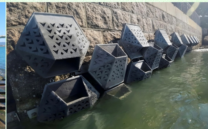
Newly installed eco-shoreline fixtures on the existing seawall in Lei Yue Mun 新設於鯉魚門現有海堤的生態海岸線組件
