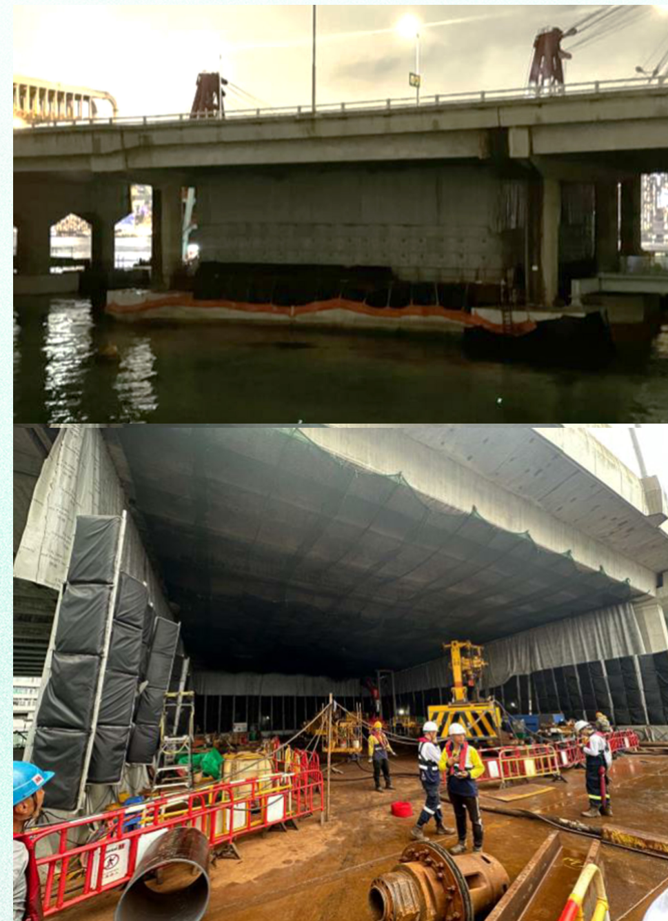
Temporary acoustic noise barrier for marine piling works near residential blocks 於住宅附近進行海上樁基工程時的臨時隔音屏障
