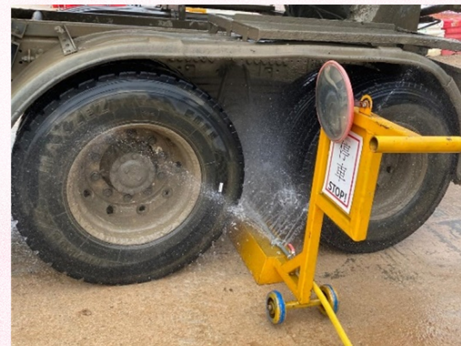
The wedge prevents the vehicle from sliding, hence also improving the efficiency of wheel washing 此楔塊能防止車輛滑動，從而提高清洗車輪的效率
