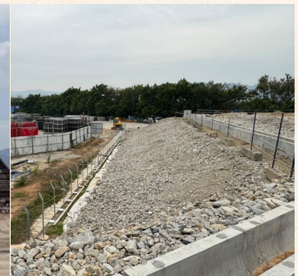
Slope built with recycled aggregates 採用循環再造石料建成的斜坡
