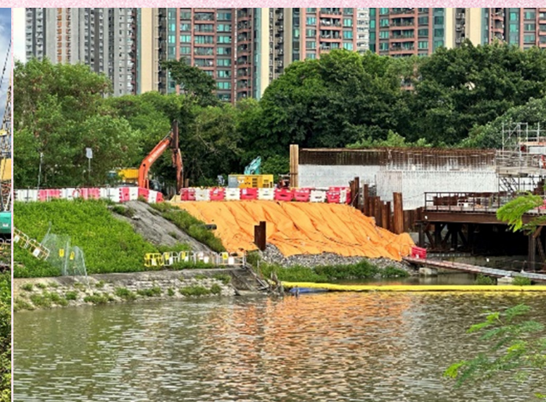
Cover the slopes adjacent to the river with tarpaulin sheet to reduce silty runoff 以防水布覆蓋鄰近河流的斜坡，從而減少泥水徑流
