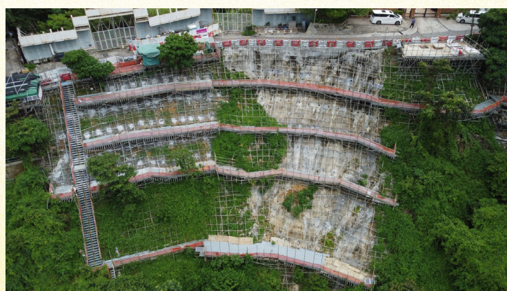
Upgrading substandard man-made slopes 鞏固不合標準的人造斜坡
