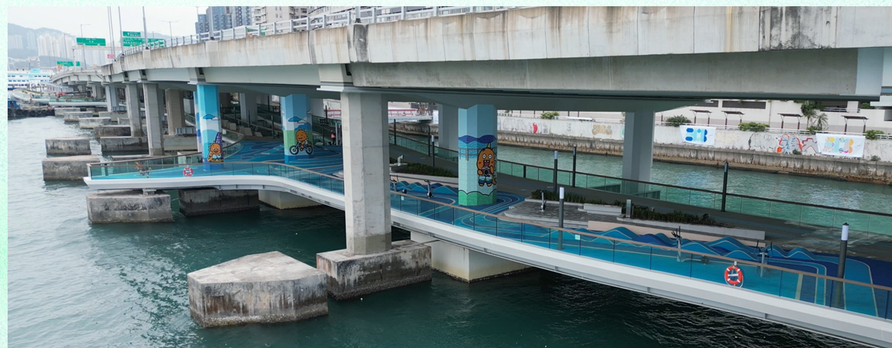
Boardwalk decks utilising existing IEC piled foundations 東岸板道利用東區走廊現有的樁柱基礎
